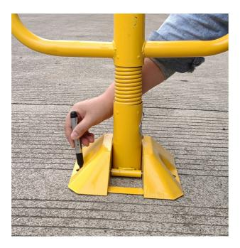
**Step 2:** Remove the lock again and carefully drill the 3 holes straight (drilling depth at least 10cm).
