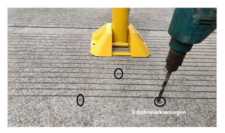
**Step 3**: Now place the parking lock base over the holes, insert the expansion bolts and tap them into the holes provided with a hammer (ideally a rubber mallet).
